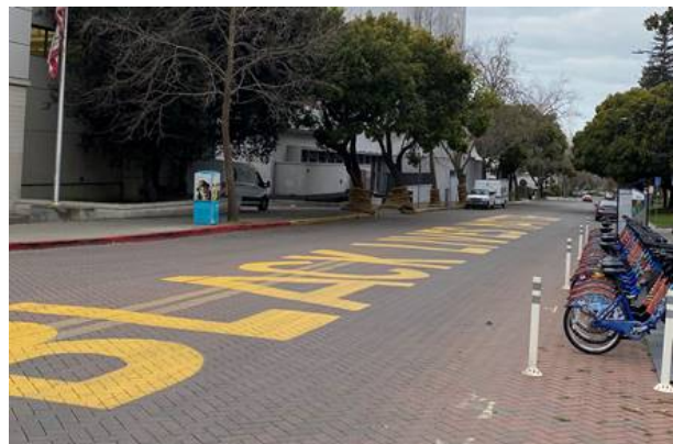
Allston Paver Project
